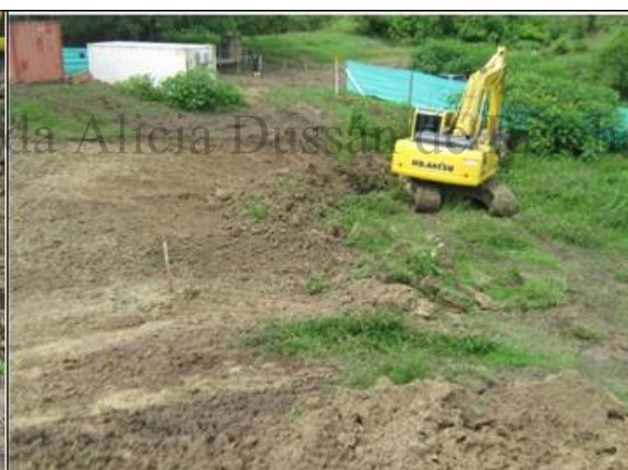
Foto 68. UMGP9 Descapote N06,48661° y W74,42113°
