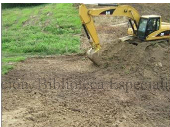
Foto 63. UMGP8 Descapote N06,48724° y W74,42042°
